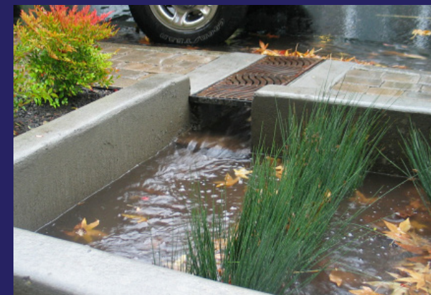
Raingardens along roadways
