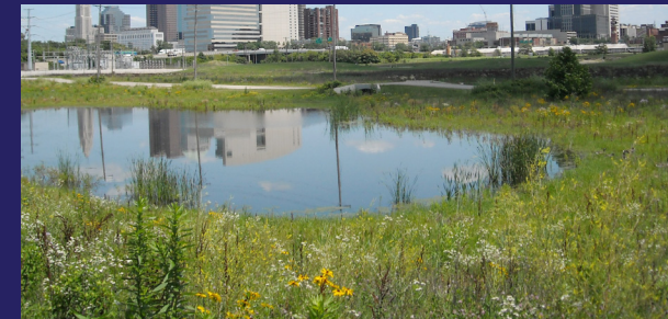
Bioswales and retention area
