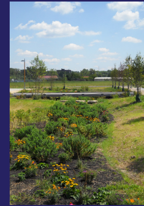
Bioswales for improved stormwater quality
