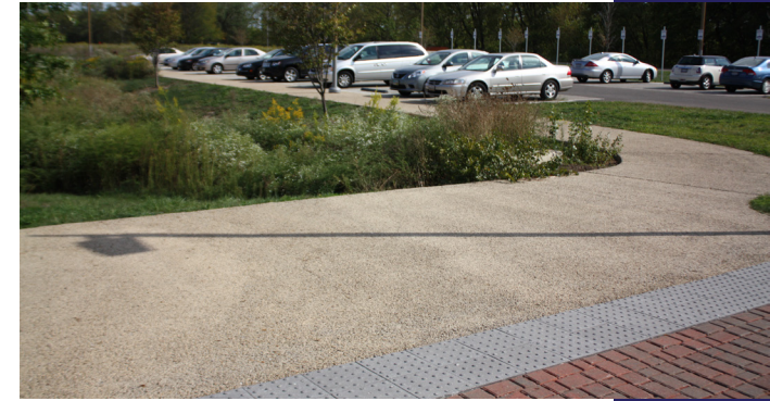
Porous pavement and a rain garden in Columbus, OH
